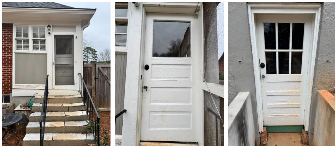
From left to right: rear exterior wall of mudroom, zoom in on rear egress door to mudroom, rear egress door to basement
