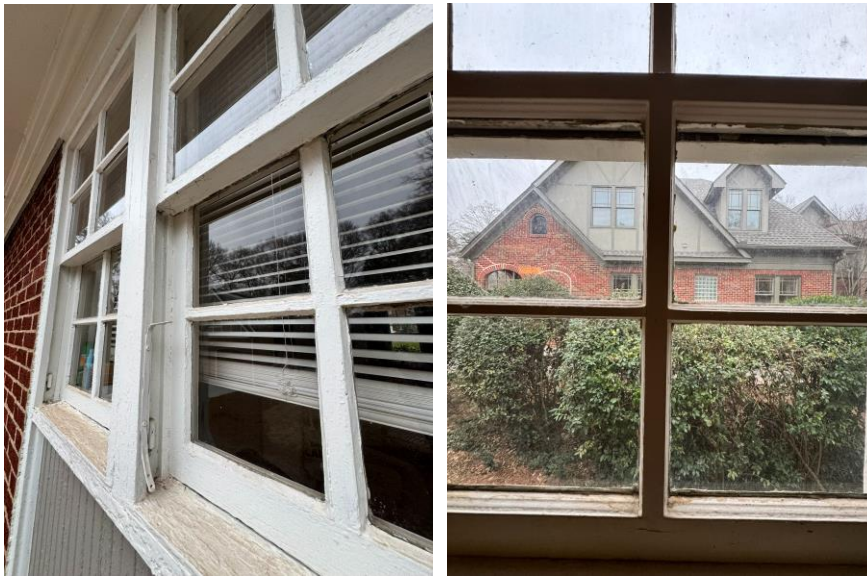
From left to right: exterior view of mudroom windows, interior view of mudroom windows
