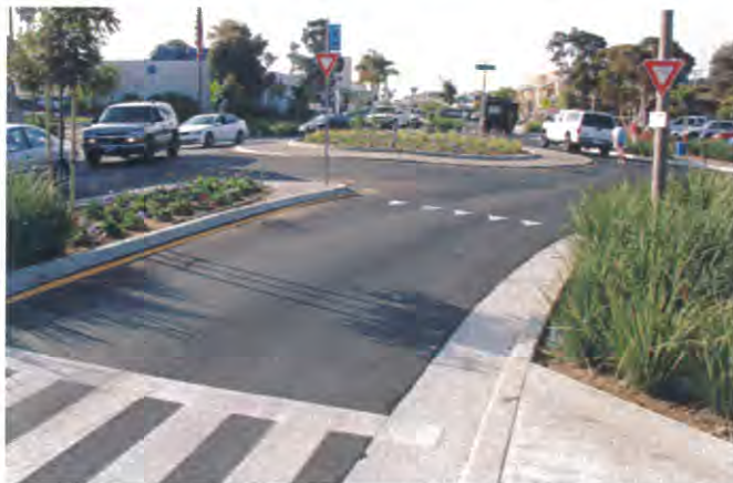
A modern, single-lane roundabout in San Diego, CA calms traffic, improves safety, and supports people walking and biking, all while carrying about 25,000 vehicles per day.
