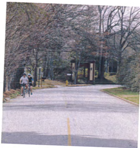
S. Avondale Road is wide enough to support a colorized bike lane heading eastbound.
