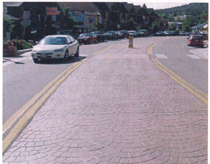
Best practice: colorized center turn lane, which allows for emergency vehicles to safely and efficiently navigate the road.
